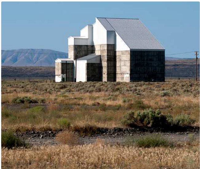
The cocooned Hanford F reactor, post-remediation
